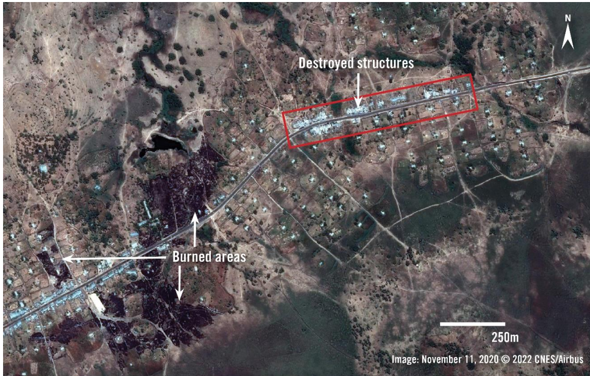
Satellite imagery from November 11, 2020 shows the eastern side of Division. Many structures along the main road are completely destroyed. According to low resolution imagery (not shown), the structures were damaged between November 5 and 10, 2020. Fires were detected in the area on November 7.
