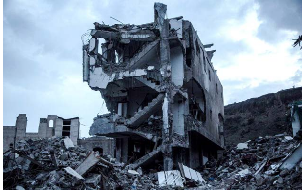
Residential building destroyed by an airstrike by the Saudi Arabia/UAE-led coalition on 25 August 2017 on Faj Attan, Sana'a, Yemen, killing 16 civilians and injuring 17 more. © Rawan Shaif
